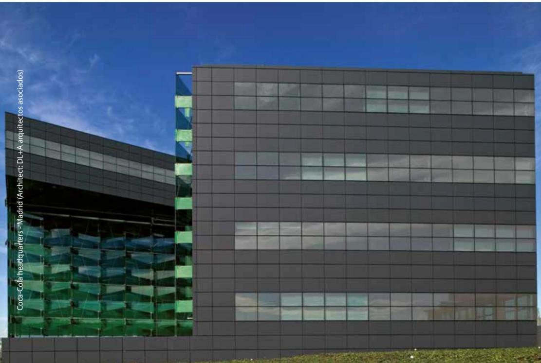
The extensive range of CW 50 profiles meets all requirements of contemporary architecture. With regard to the thermal performance, the system offers solutions in different levels, allowing the use of triple glazing and making the system even applicable for passive house or low energy buildings.
